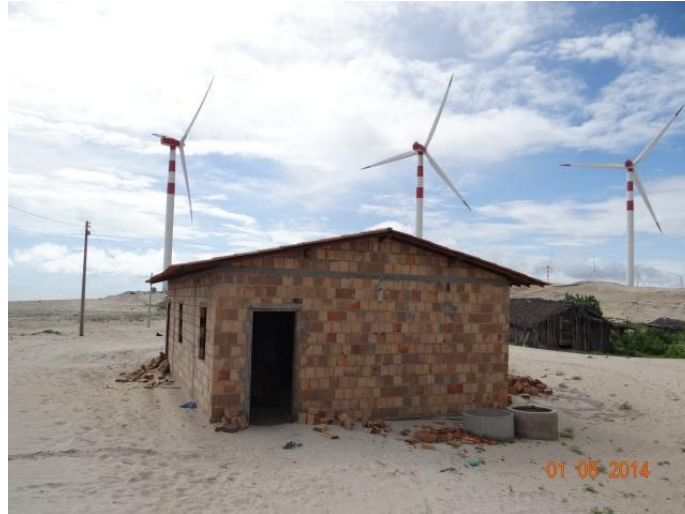
Figure 12: Brick house in construction in Xavier community. Source: Jocicléa Mendes (2014)
